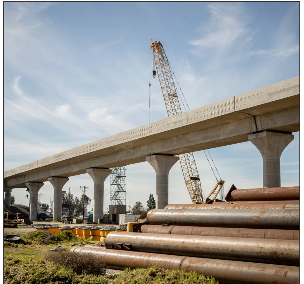
Construction on the high-speed rail project above Highway 99 in south Fresno on March 6, 2023. Photo by Larry Valenzuela, CalMatters/CatchLight Local
